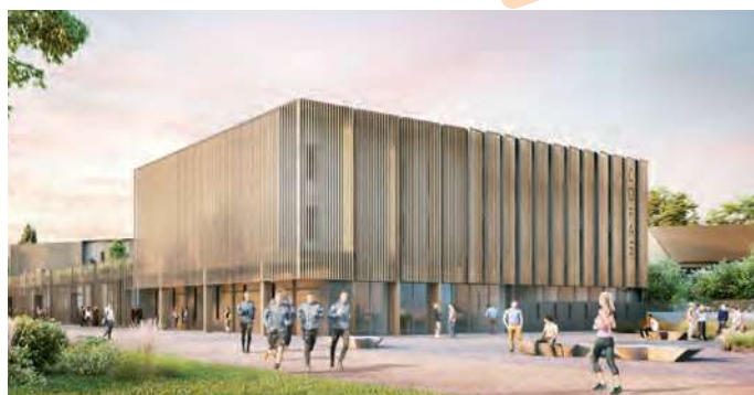
Extension du cdfas - credit Atelier 234
